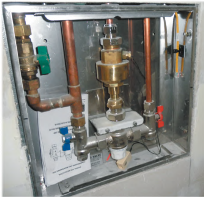
Image 2 – TMV Monitoring system typical installation.
