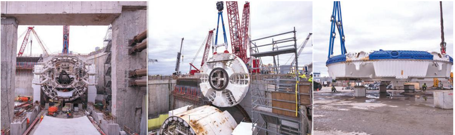
[LEFT TO RIGHT]: 2 A view of the TBM shield from the first trailing gantry. 3 The TBM cutterhead is lowered into place. 4 Cranes lift the TBM cutterhead so crews can remove the concrete support blocks. 5 The crane swings the TBM cutterhead into position over the launch pit. 6 VDOT Project Director Jim Utterback and HRCF Project Manager Louis Brais take a minute to celebrate the progress.
