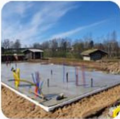
Slab foundation (with floor heating)
