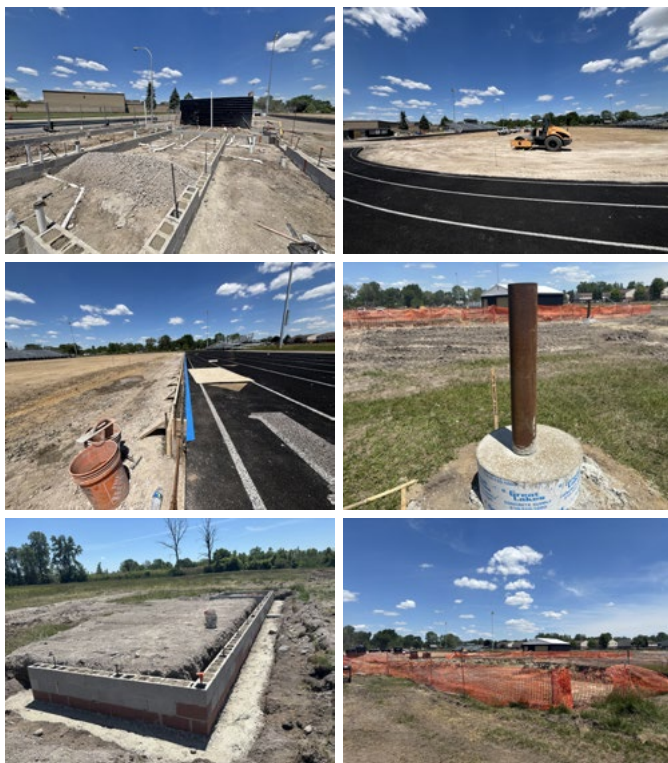
Taylor High School Athletic Complex construction includes: concession and toilet rooms (top left) and the football field (top right); installation of a concrete turf anchor (middle left) and backstop foundation (middle right); and completion of the dugout foundation (bottom left) and excavation for underground stormwater storage required by the county (bottom right).
