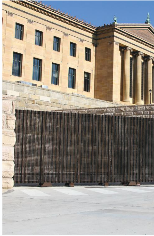
Right: Box Frame Roller Gate, Clear opening width 60 feet 2 inches by 10 feet high, Pg. 18
