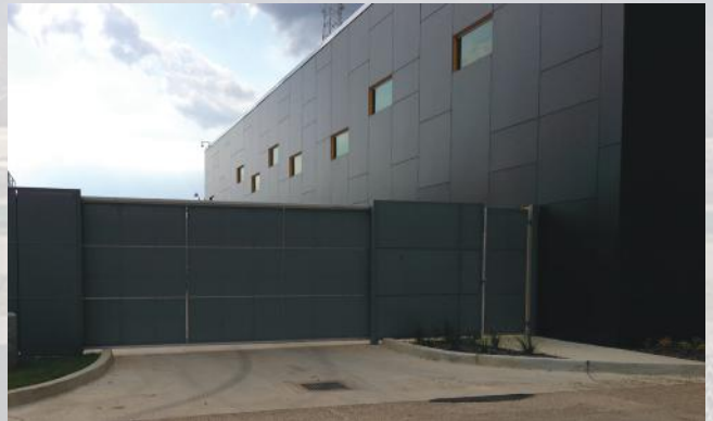
Right: Structural Cantilever Gate.
