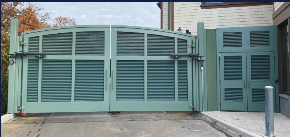
Right: Belmont Retail Village, NY Custom Swing Gate System.
