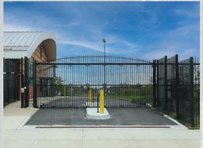
Right: Structural Cantilever Slide Gate.
