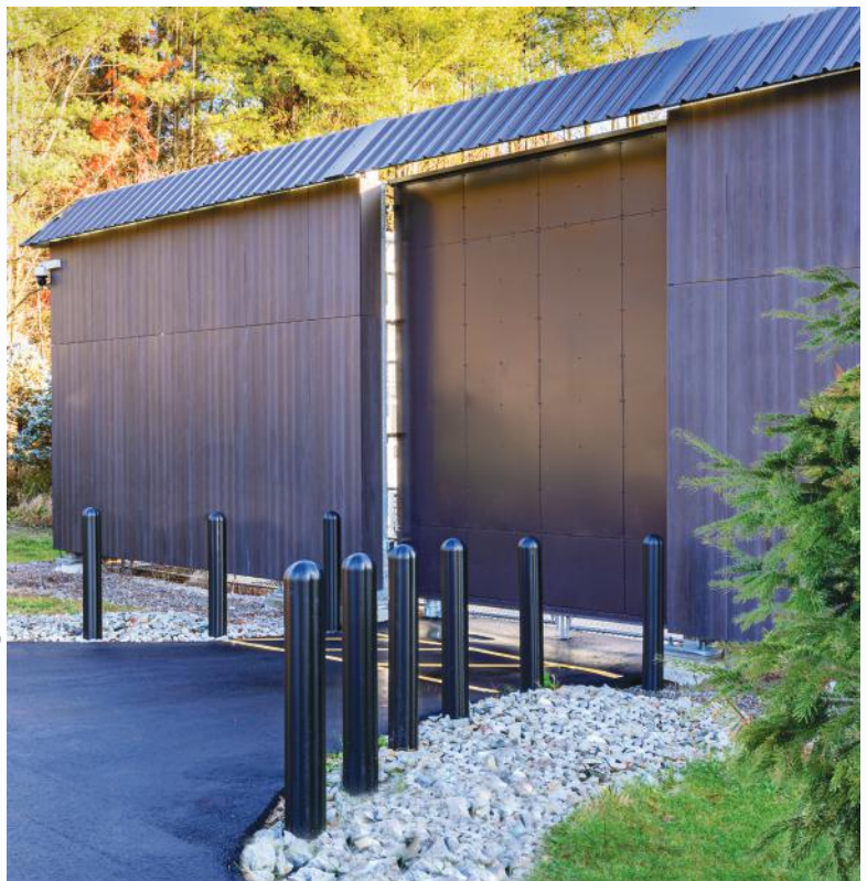
Right: Eversource Sharon Substation, Custom Structural Cantilever Gate. Pg. 14
