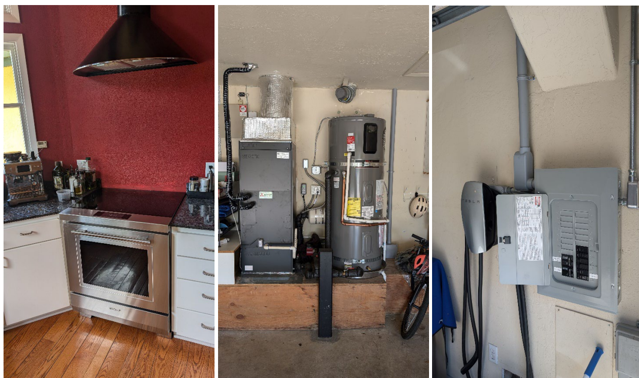
Figure 7: The new electric induction stove, the heat pump air handler and heat pump water heater, and the electric car charger next to the subpanel for the water heater.
