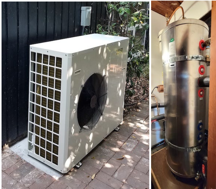
Figure 9: The outdoor Chilltrix hydronic heat pump and in the inside buffer water storage tank.
