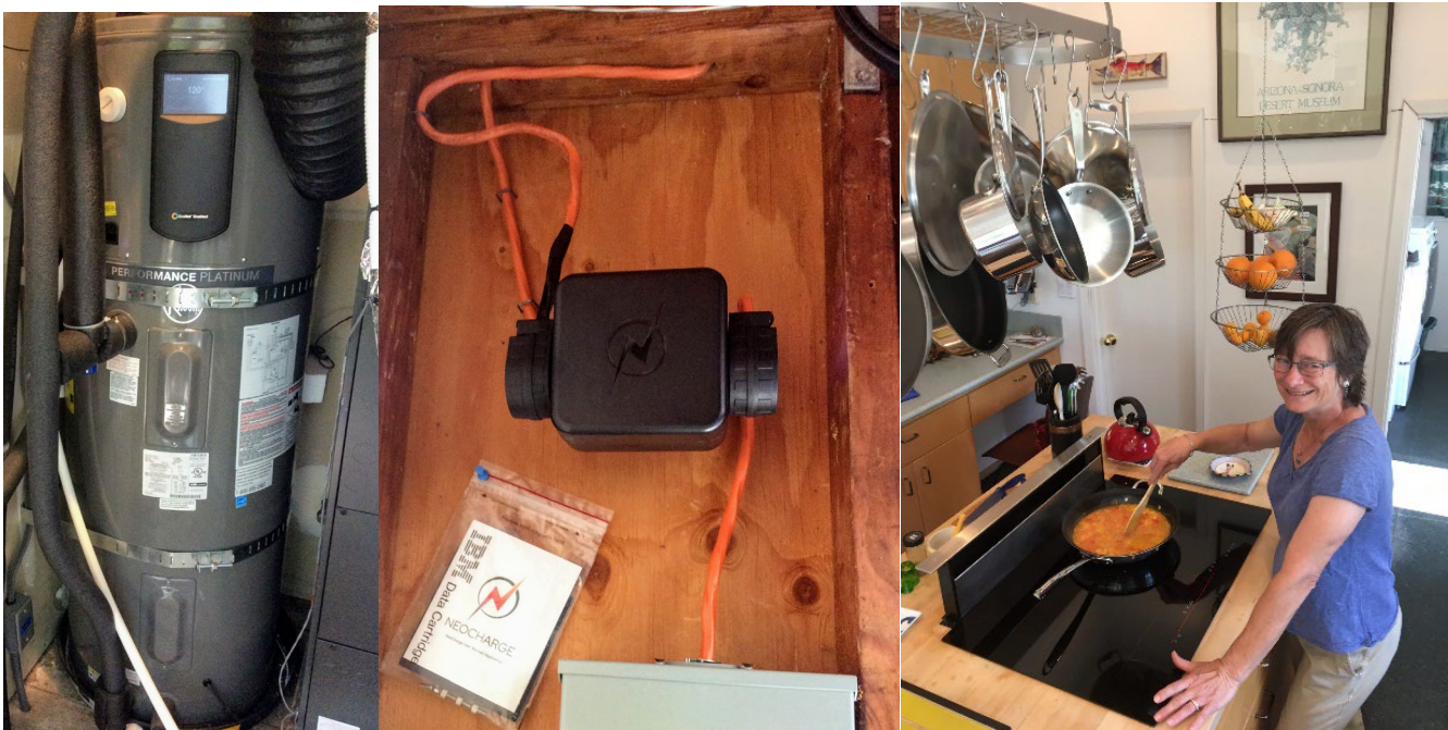
Figure 14: At the Schmidt’s home, the Bosch electric induction stovetop 26 is shared on the same circuit as the Rheem heat pump water heater 27 using the NeoCharge (middle) (Images courtesy of Steve and Lisa Schmidt).
