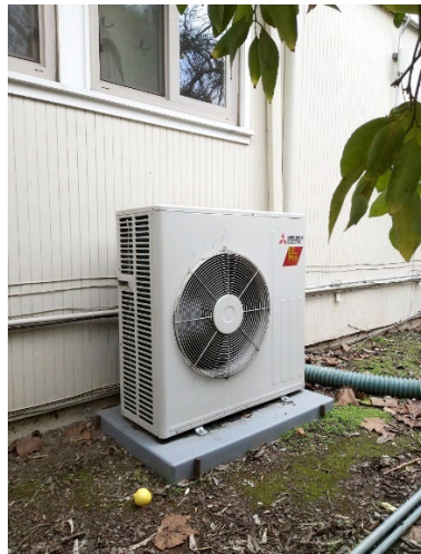
Figure 12: The min-split heat pump outdoor and indoor units.
