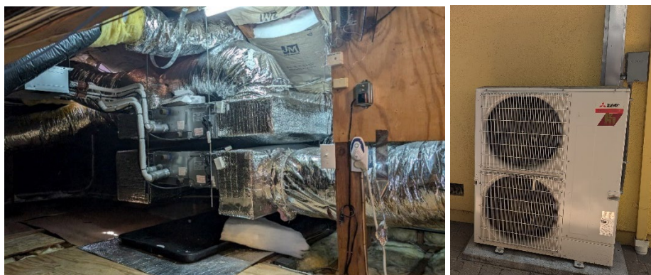
Figure 8: The heat pump air handler in the attic, and the heat pump compressor sitting on the outside of the house.
