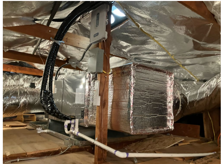
Figure 4: The new HVAC system installed in the attic, with ample insulation around the heat pump itself, and on the lining of the rafters.
