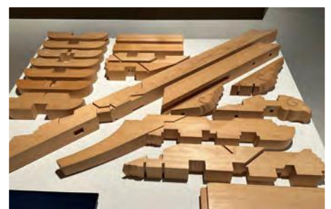
▲ Examples of kigumi (joinery) techniques that produce precise, interlocking sections, which do not rely on metal or nails for strength
