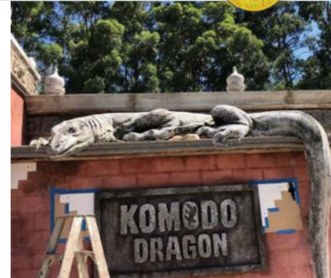
Installing the lizard sculpture
