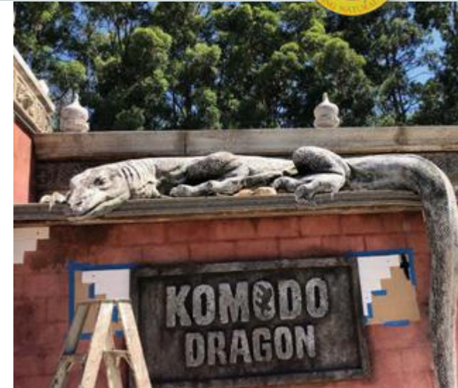
Installing the lizard sculpture
