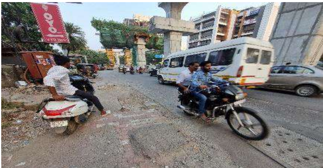
Figure 4: Image of Road Conditions
