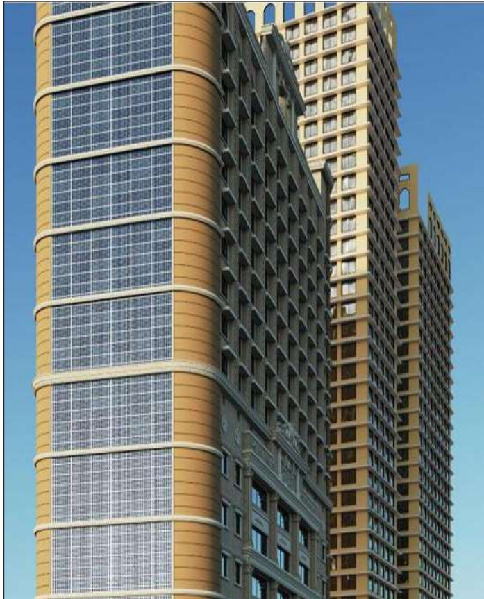
Figure 2: AL – Rehan Building Mumbai
