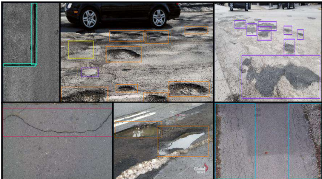
Figure 2: Annotated Images: Cracking (Red), Alligator (SkyBlue), Pothole (Orange), Patching (Violet), Ravelling (Yellow), Sealing (Light Green)
