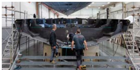
Maxi deck installation.
