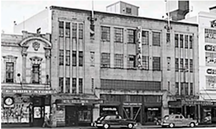
Todd Motors building, which once stood where the derelict Reading cinema complex is now. Photo: digitalnz.org.
