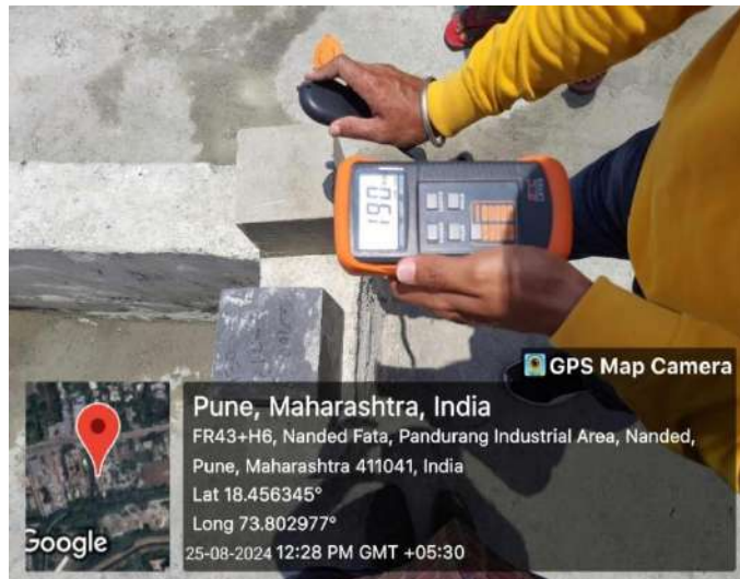
Figure 5: Concrete Block (Conventional)
