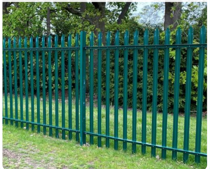
Metal Perimeter Fencing
