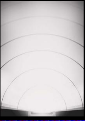
Typical light spill from flood light
