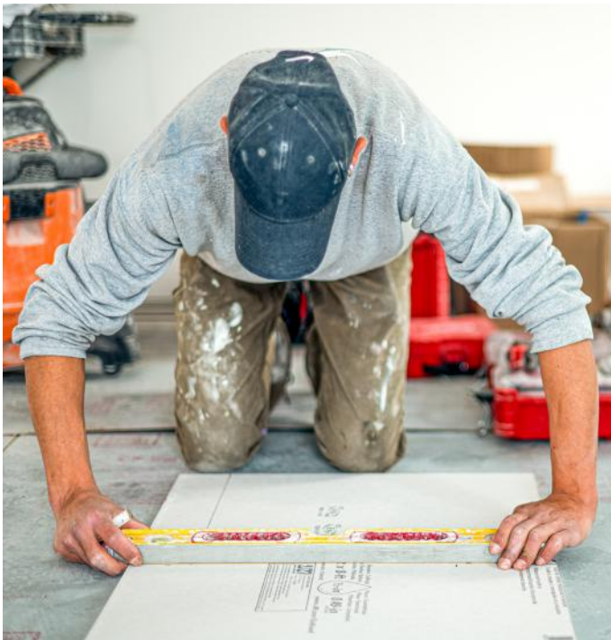
Sal Azzolino of Argo Tile & Stone in San Francisco, measuring and cutting GoBoard to fit.
