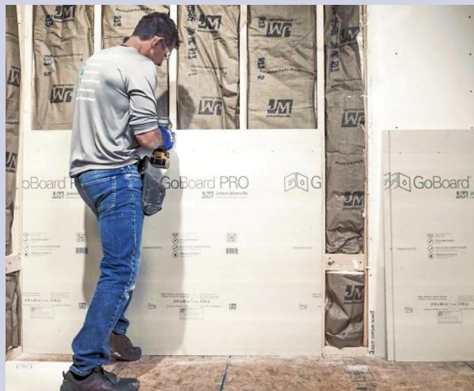
Matt Wentland, a Colorado general contractor, installs GoBoard PRO.
