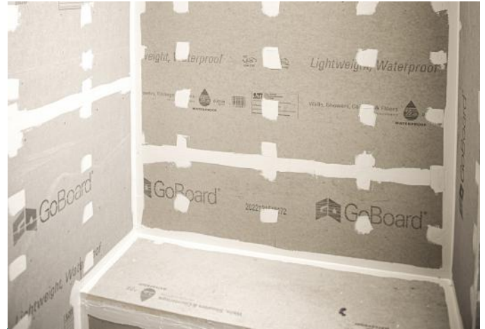
A GoBoard shower installation by Brandt Garrison in Burley, Idaho.
