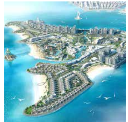
QETAIFAN ISLAND NORTH, QATAR Featuring GEBERIT & BOSSINI
