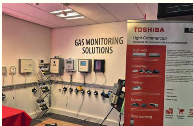
Inside the new Wakefield training centre
