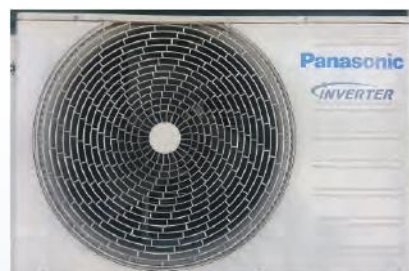
R410A split air-conditioning unit converted to RS-53 (R470A) & operating satisfactorily without any problems
