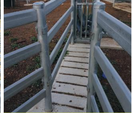
Concrete Work Areas
