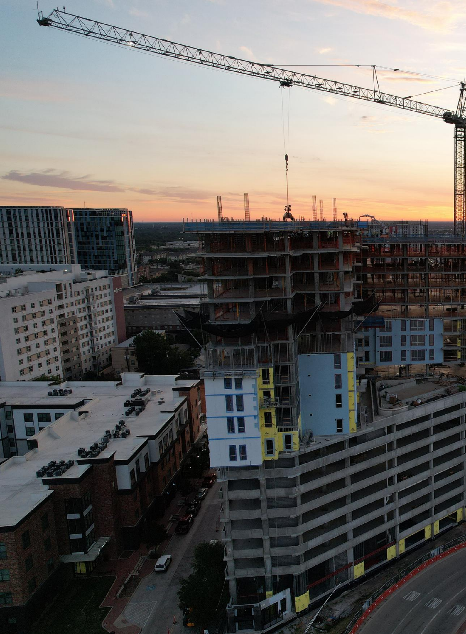
Up Campus - College Station, Under Construction 2025
