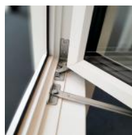
Handle operated brake
