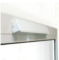
Trickle vent - Exterior
