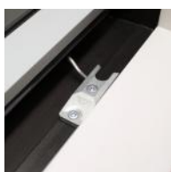
Handle operated night latch
