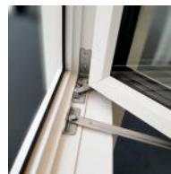
Handle operated brake
