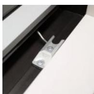
Handle operated night latch
