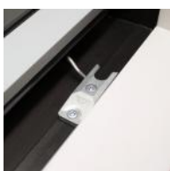
Handle operated night latch
