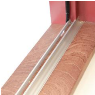
Hardwood threshold Inward opening door
