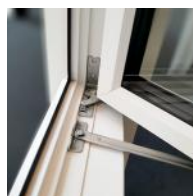
Handle operated brake
