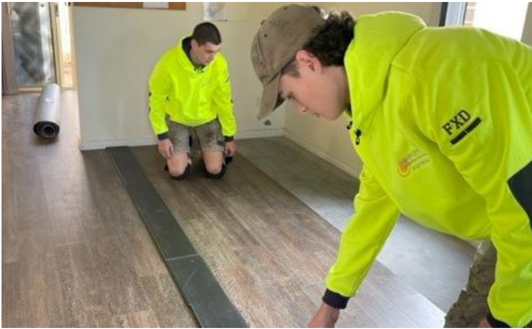
Bryce and Heath laying planks provided by Karndean
