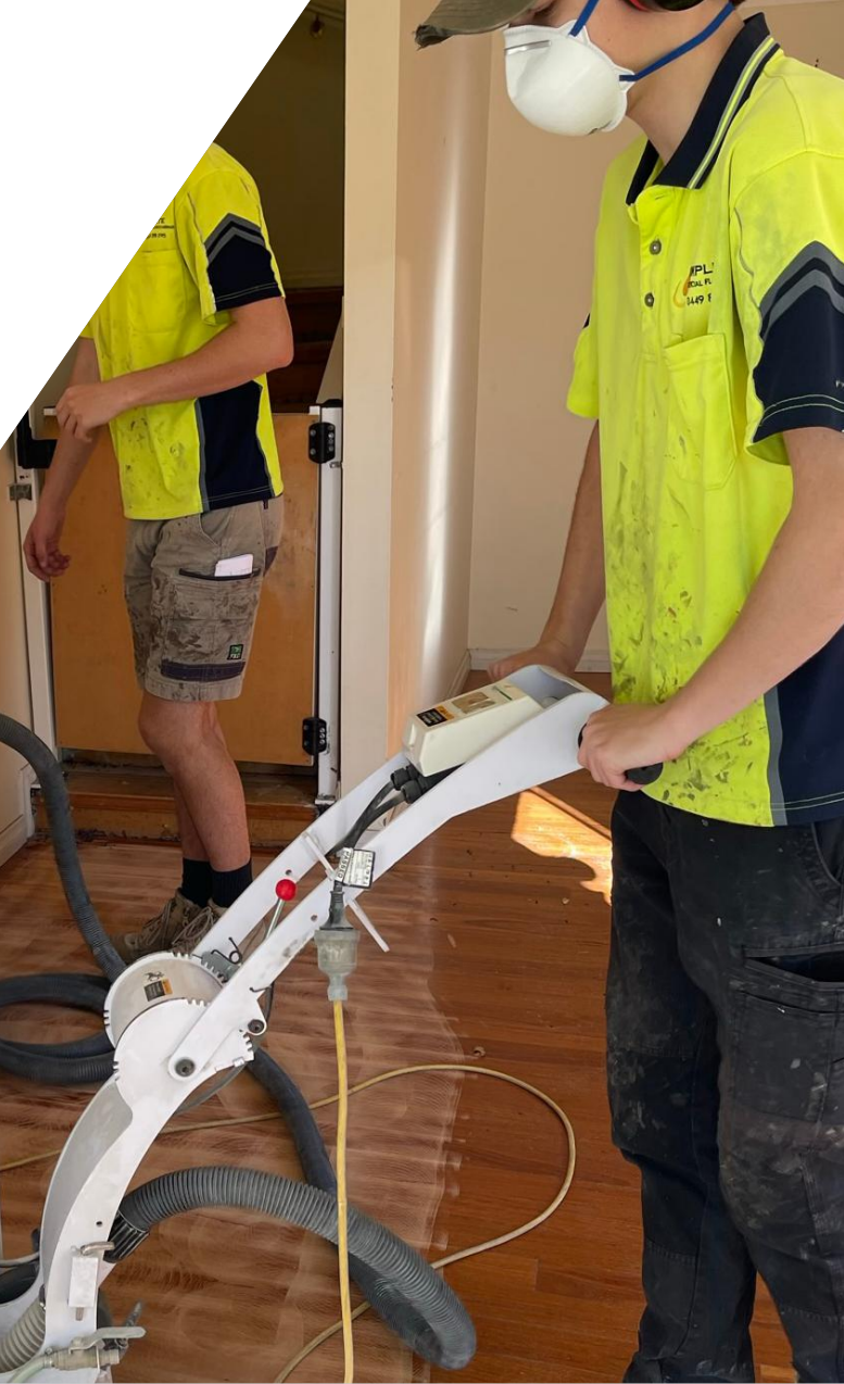
Heat grinding the subfloor at SAHSSI workshop
