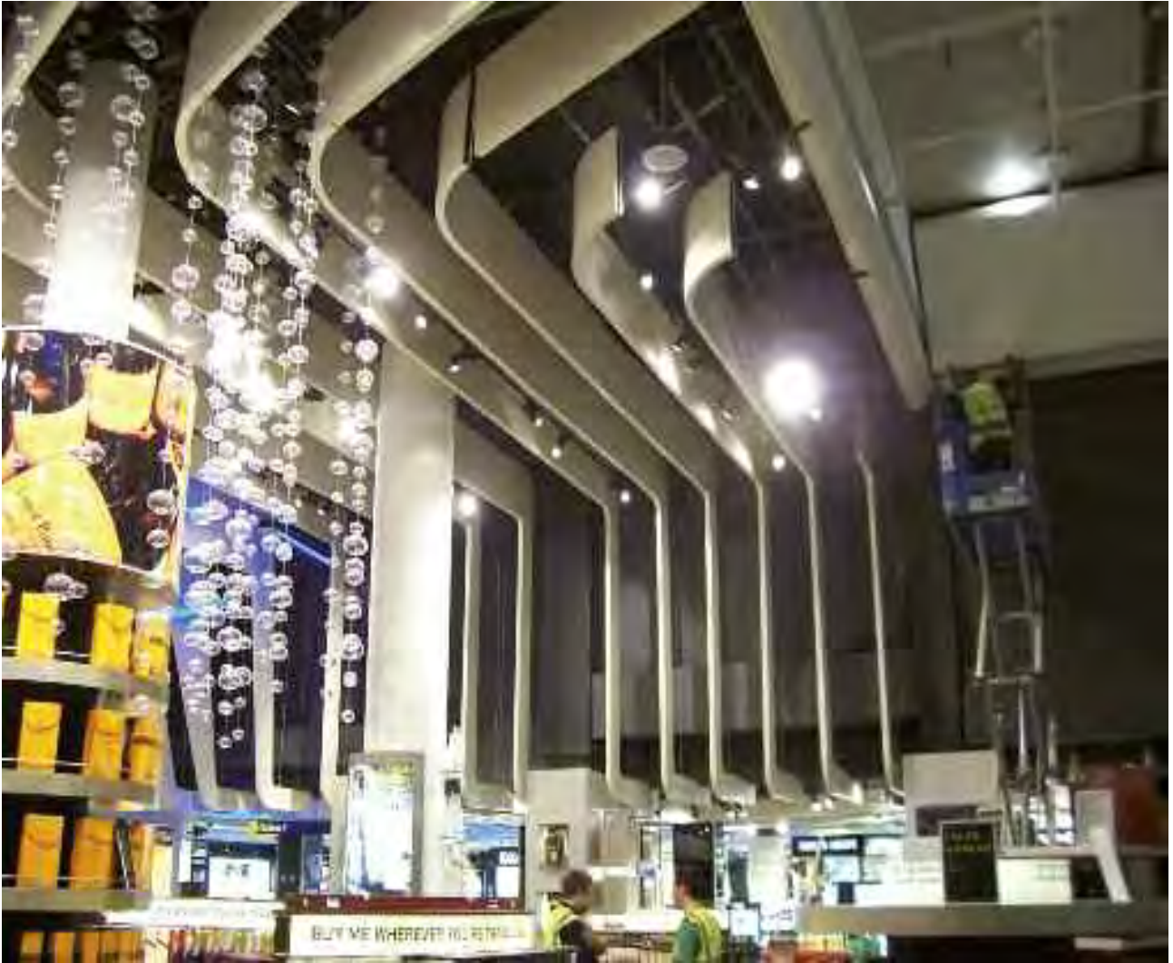
Project : Manchester Airport T1, Biza Retail (Tax&DutyFree) Location : Manchester, United Kingdom Product : Quadroclad® Baffles (straight, curved, special shapes) Architect : Christopher Hampshire
