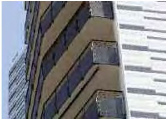
Project : Joaquin Turina Apartments Location : Barcelona, Spain Product : 150F Architect : Enric Perez and Joaquim Ballarin
