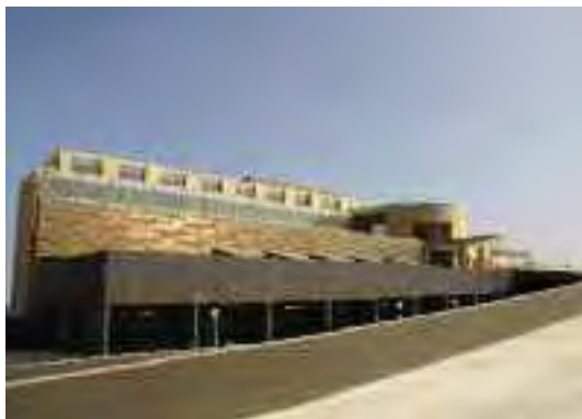
Project : Hotel del Desierto de Enjoy Antofagasta Location : Antofagasta, Chile Product : Screenpanel in Copper Architect : Estudio Larrain
