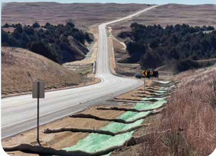
Asphalt Paving - Tryon to Mullen
