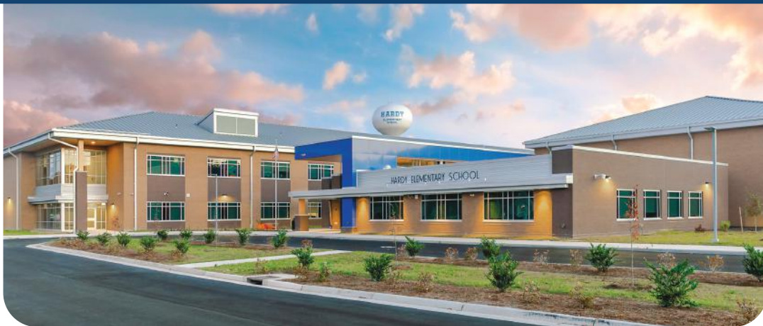
PHOTO COURTESY OF IWCS
