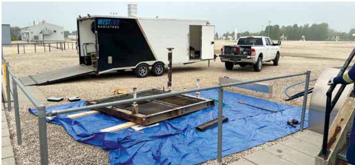
West End Radiators' mobile technicians repair a back-up generator heat exchanger on-site.
