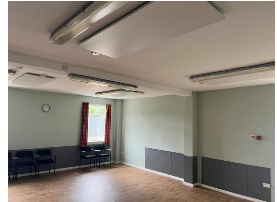
Example village hall now insulated, with infrared panels suspended from the ceiling
