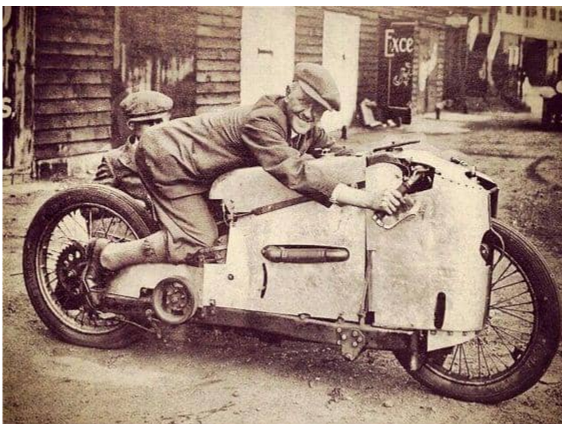
"George and the giant. GH Tucker demonstrates the curious kneeling position which he adopts in riding the new supercharged four-cylinder AJW. The small wheel just below the rider's knee is the drum of the transmission brake."
