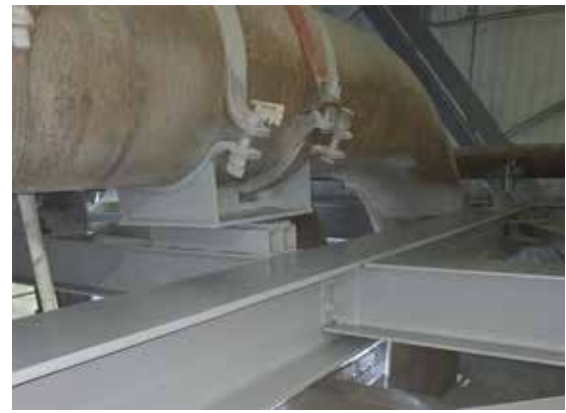
ICE Dragon Corrosion has supported many mining operations from the design phase through construction/commissioning and into operation and maintenance.
