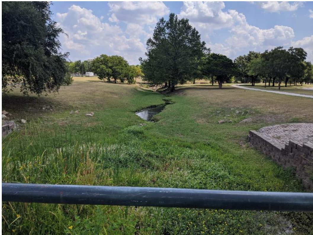
Figure 2.1 – Field survey location at Bull Branch & Davis Street
