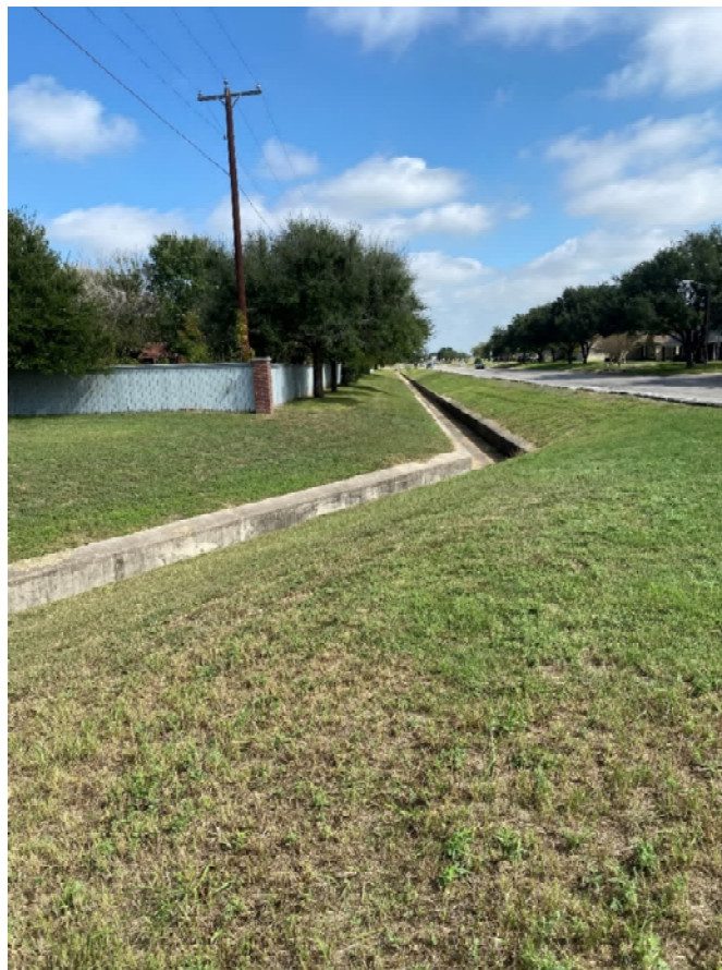
Figure 3: Concrete drainage channel entering pond, looking east
