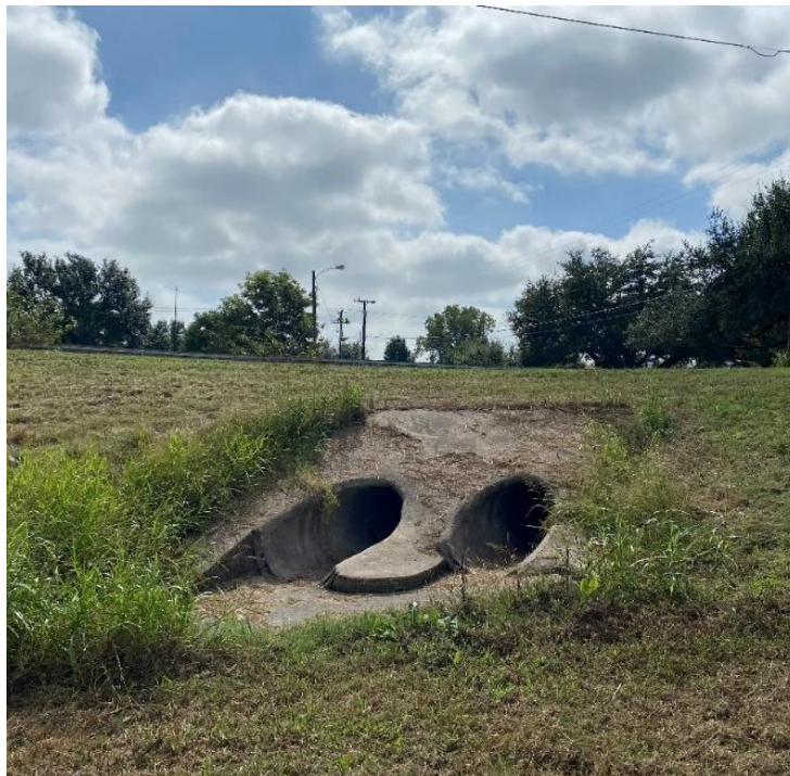
Figure 1: KBI Pond principal spillway: two 36-inch RCP
