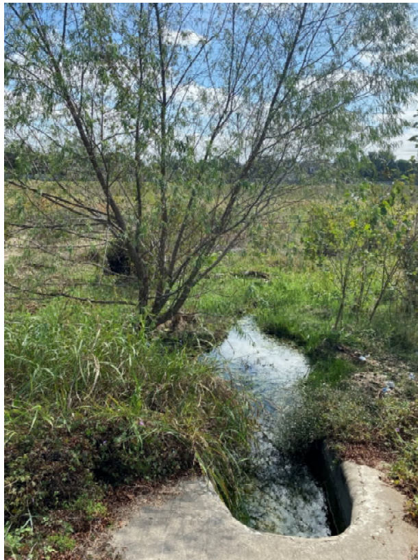
Figure 5: Pond inlet adjacent to depression with standing water
