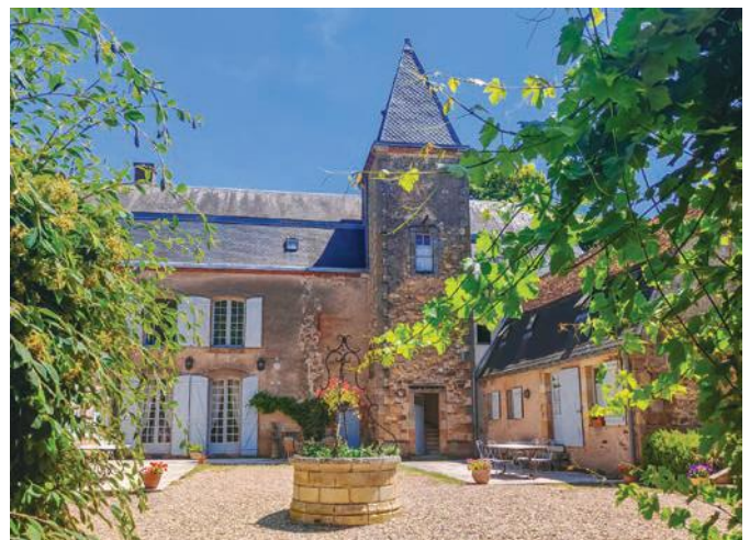
The central courtyard has access to the private guest wing and kitchen
