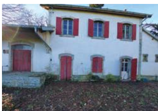
€120,000, Valzin-en-Petite-Montagne, Jura: With grounds and views, this three-bedroom former railway station requiring work is 15 minutes from Vouglans lake (Thomas Lugand, IAD France)
