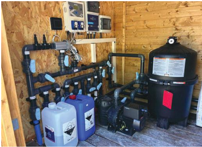
A new cartridge system with a variable speed pump is cost-effective
