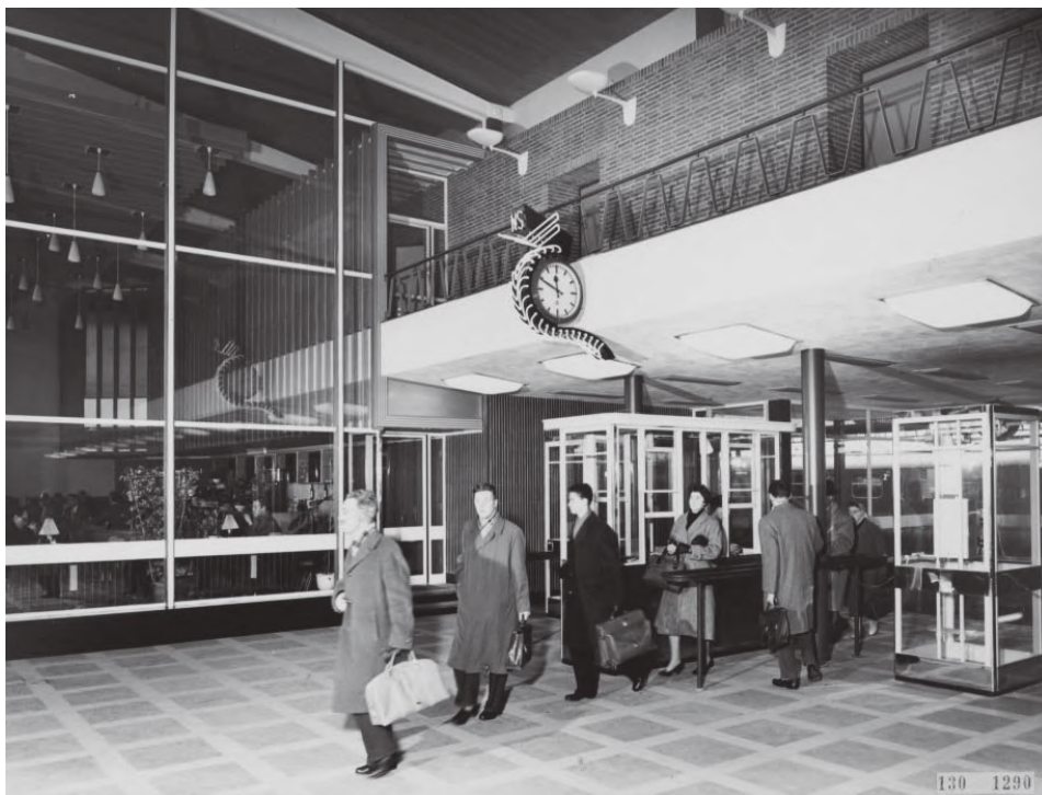
Centrale hal, ca. 1960
