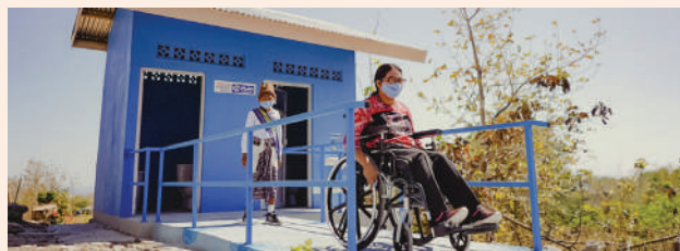
Construction of proper, gender-equal, and inclusive toilet and sanitation facilities in West Nusa Tenggara and East Nusa Tenggara. These toilets are equipped with handrails, toilet seats, hand washing with soap (HWWS) facilities with a certain height, and Menstrual Hygiene Management (MHM) facilities.
