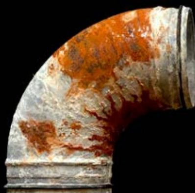
Unreated substrate Unwashed
