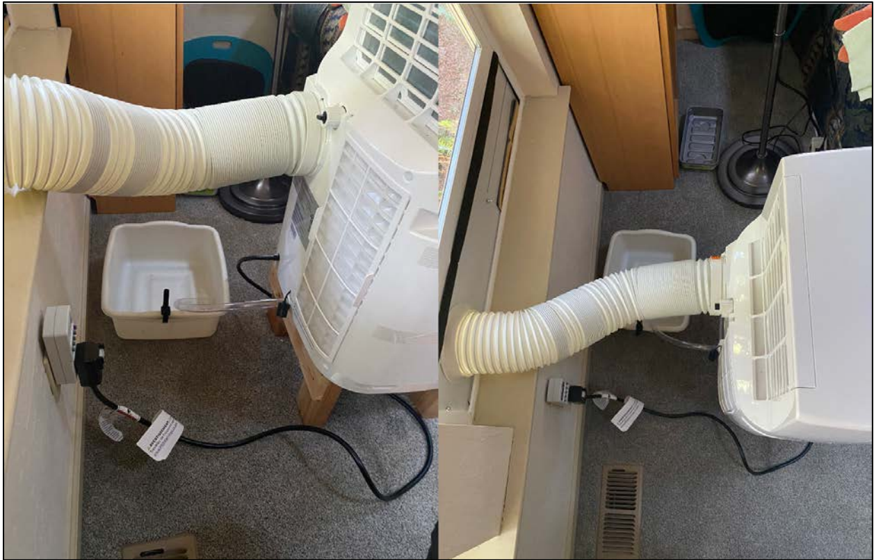
Figure 5: Back view of the Honeywell unit showing the single exhaust system connection and the water bucket installed for condensation to drain in. The heat pump does not come with a water pump that could pump the water outside, so only gravity was used.
