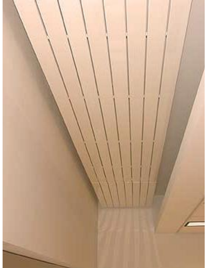
Radiant Ceiling panels installed linearly show they are both a utility and architectural feature.
