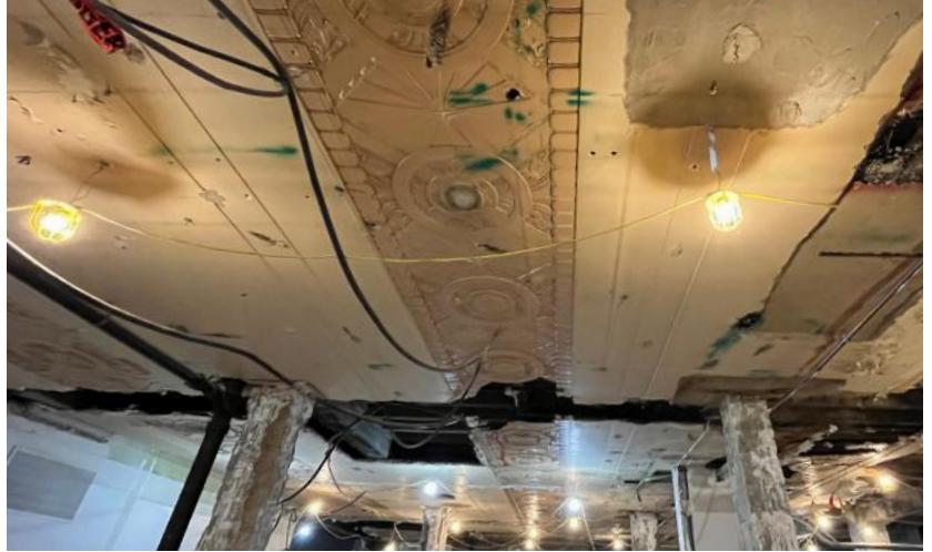
Detail of the Historic Lobby Ceiling.
