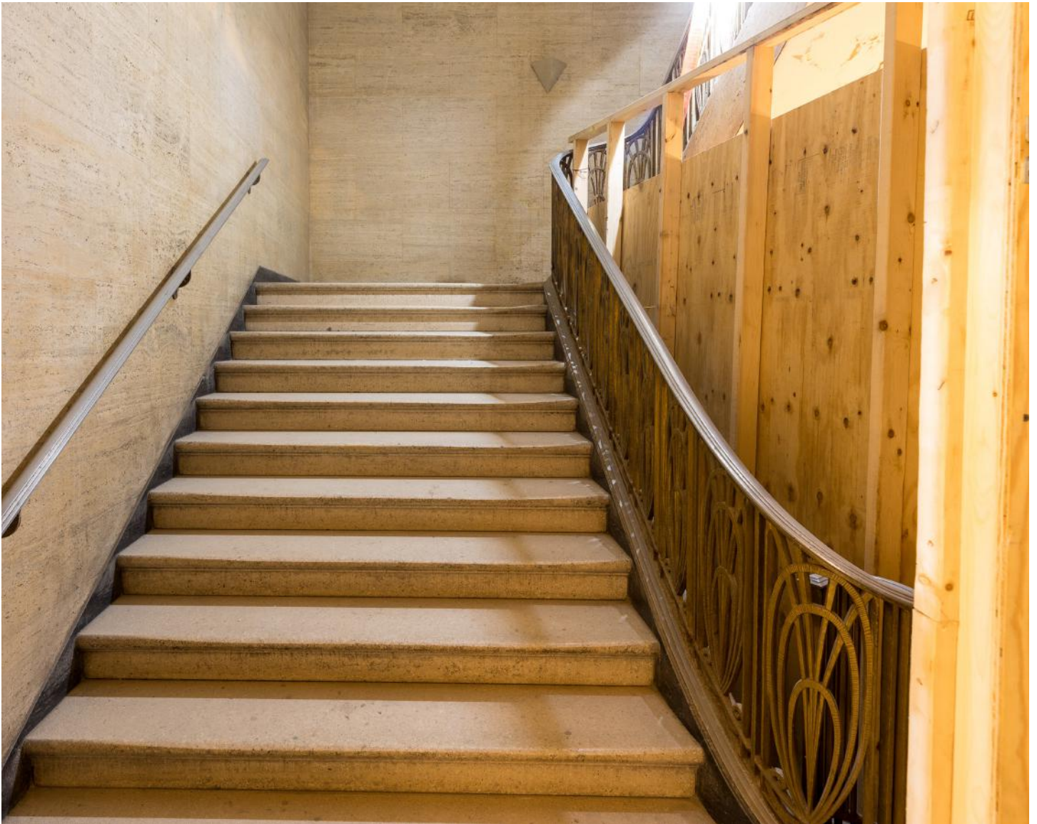
Details of the Historic Central Stair and construction in-progress.
