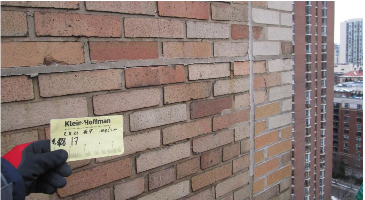
Klein & Hoffman verifying existing conditions of the façade.
