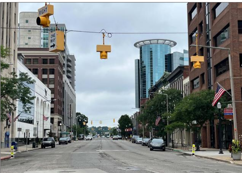
FIGURE 17: E. Michigan Avenue "Before" In 2022, the one-way downtown street was wide, unsafe, and unused by pedestrians.
