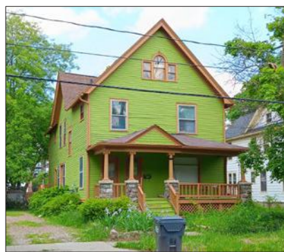
Existing Kalamazoo Duplex in the Vine Historic District
