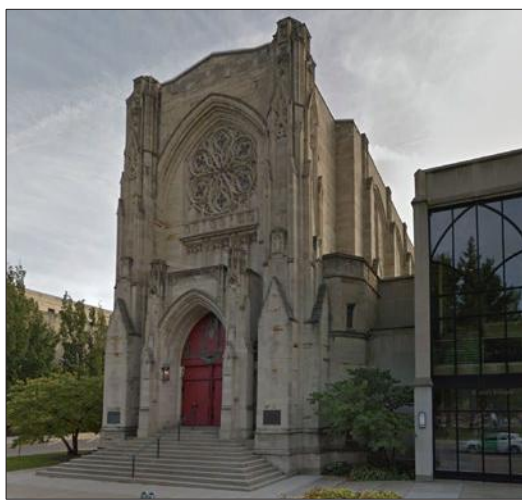
First Presbyterian Church Source: Google Street View
