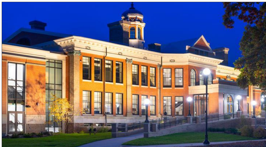
Renovations to East Hall, Western Michigan University Source: Adobe Stock
