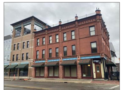
A row of historic mixed-use buildings on Pitcher Street
