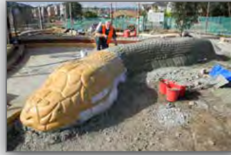
First Coat of Paint being applied - - Image 3
