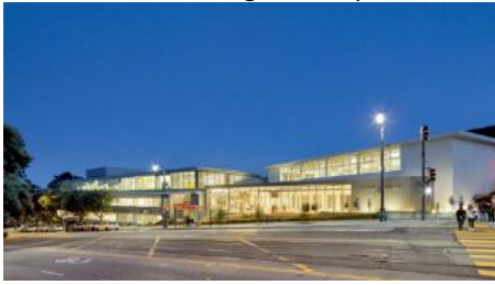
Lick Wilmerding High School 55,000 SF Architect: EHDD MEP: Integral Group
