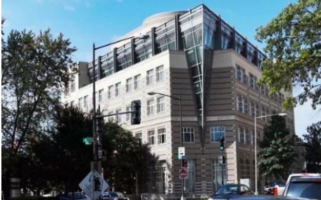
American Geophysical Union Interface Engineering
