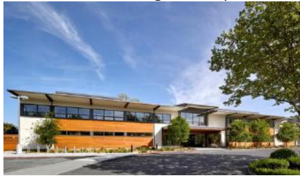
Mark Day School 14,574 SF Architect: EHDD MEP: Integral Group
