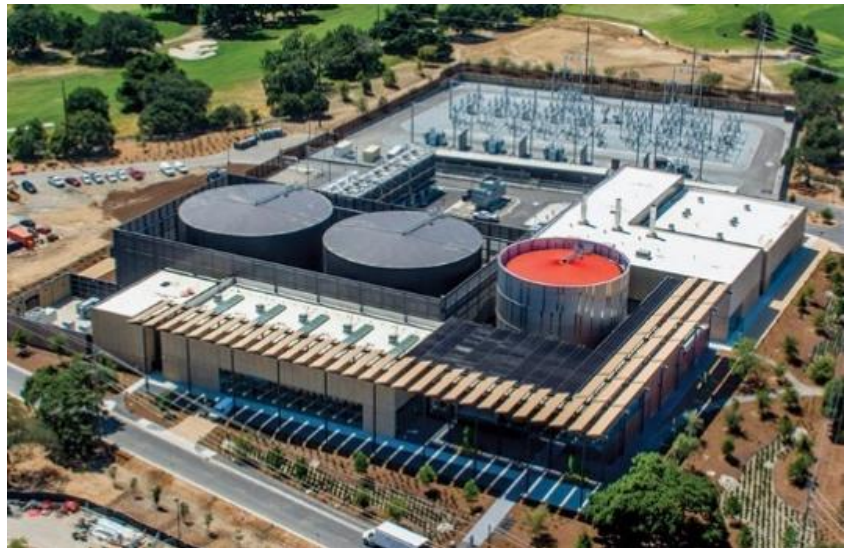
Figure 5: Stanford University's Central Energy Facility of water source heat pumps and heat exchangers.
