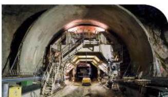
TUNNEL CONSTRUCTION & MAINTENANCE
