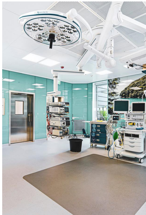
Image: Lower Queen Street Health 2 Fit-out
