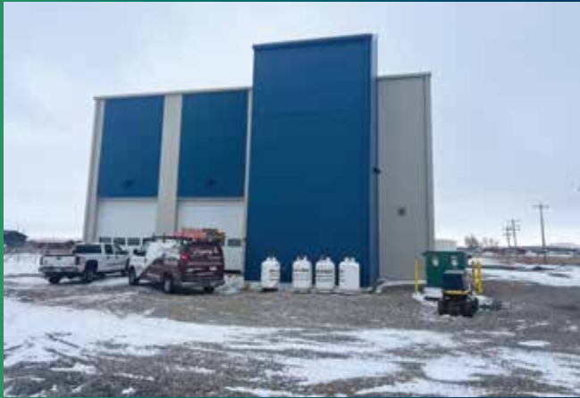
Piikani Fire Hall, Southwest Design & Construction.
