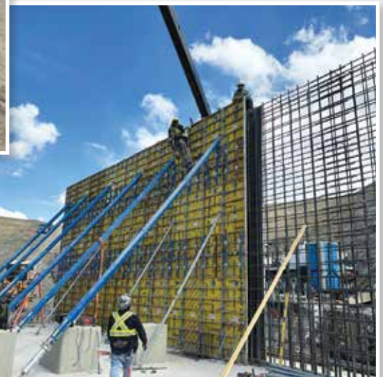
SMRID Chin Chute Replacement. VHL Construction Ltd.
