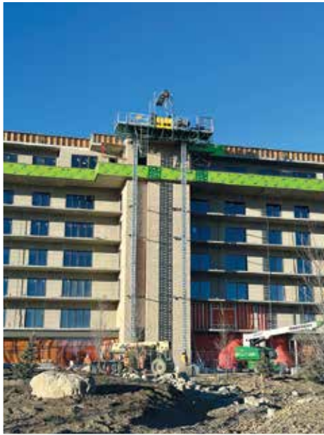
102 Scenic. Titan Masonry Ltd.
