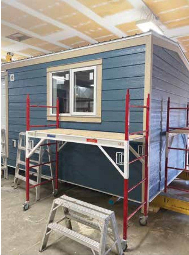
90 per cent of BTEST graduates secure employment within a week of completing the course, often in carpentry, building maintenance, or custodial roles.
