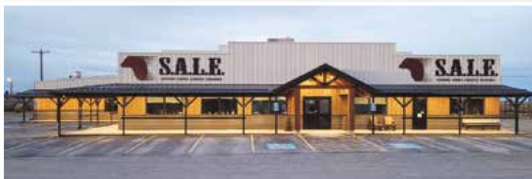
Southern Alberta Livestock Exchange new office addition. Link Builders
