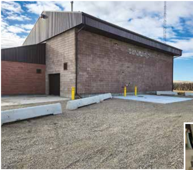
Brocket Water Treatment Plant upgrades. Nitro Construction Ltd.
