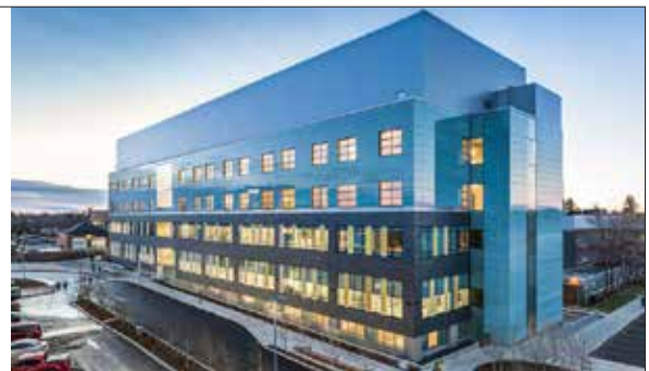
Chinook Regional Hospital Renovations
