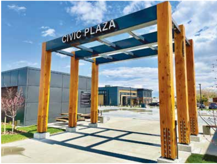
Coaldale Civic Square. Bel-Aire Welding Ltd. 2025
