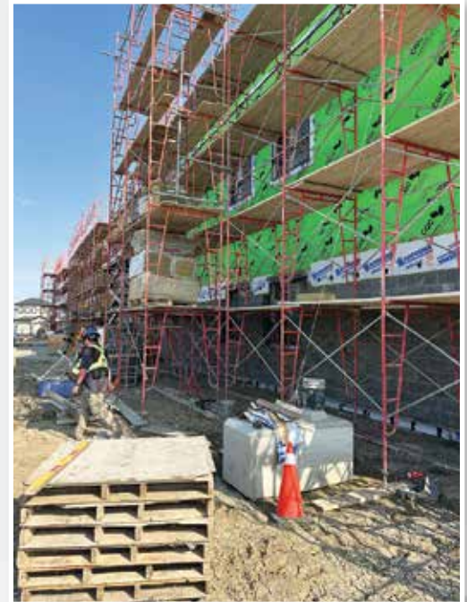
Garry Station. Titan Masonry Ltd.
