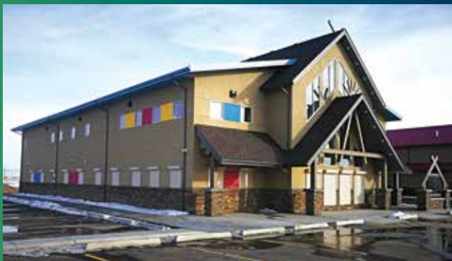
Kainai Wellness Centre, Nitro Construction.
