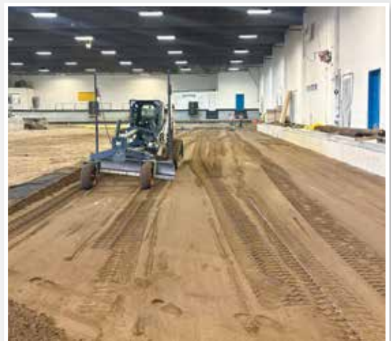
Vauxhall hockey and curling rink slab replacement. Link Builders
