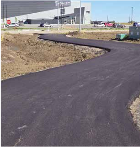
Path to new Prairie Winds Secondary School & Shift Community School. Ground Breakers Construction Ltd.
