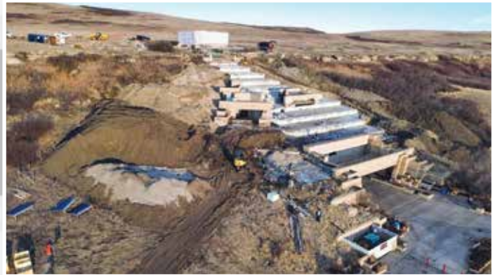
Buffalo Jump membrane replacement. Nitro Construction Ltd.
