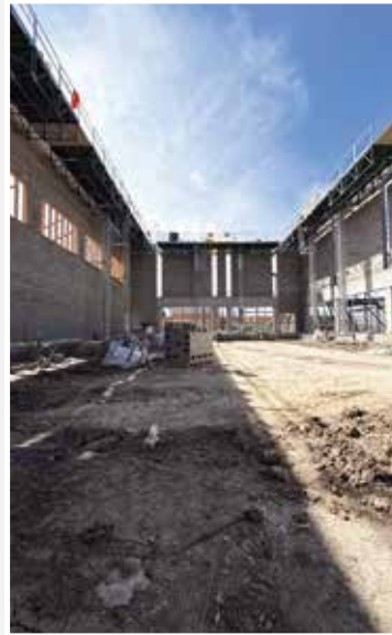
Piikani Nation K-12 school in Brocket. Titan Masonry Ltd.
