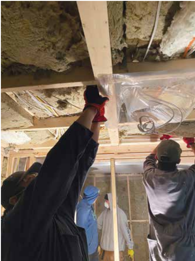
On the Blood Reserve, BTEST's graduates are contributing to local construction projects, including housing developments and community infrastructure.
