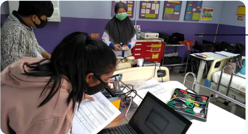
Planned Preventive Maintenance (PPM) at Klinik UiTM
