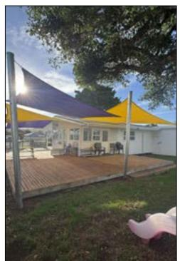
145x40mm timber beams. The lower sail edges were secured with custom roof brackets installed into the corrugated iron roof. The overlapping design allowed for a practical solution that shaded the deck that had been to hot to walk on for the children while keeping the sail size under 50sqm and adding a feature design to the centre.
