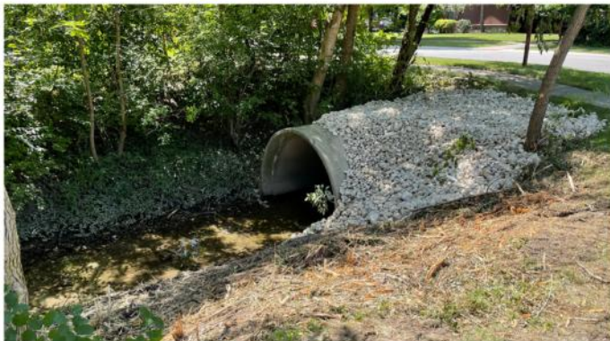
A survey of all drainage ditches within the City was completed.
