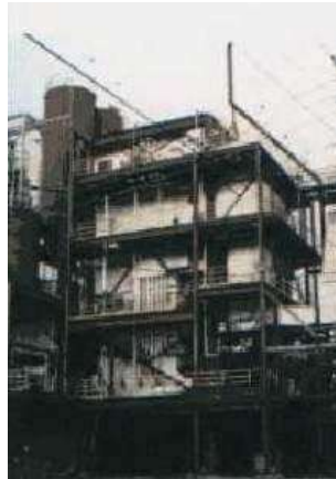
Field Erected Boiler With Superheater
