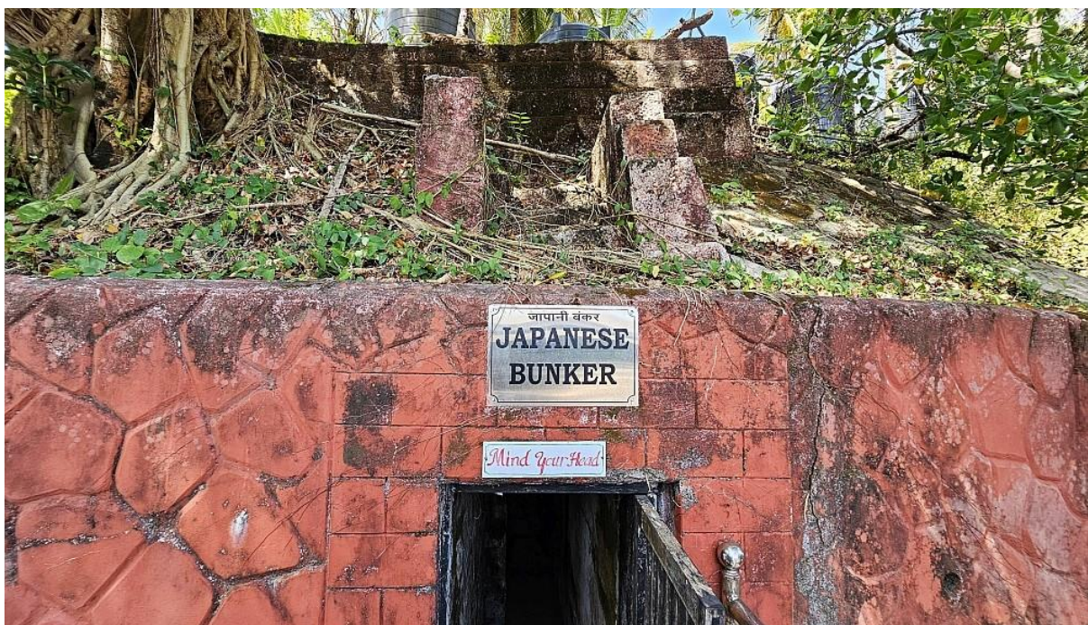
A Japanese bunker built inside the Chatham Saw Mill premises
