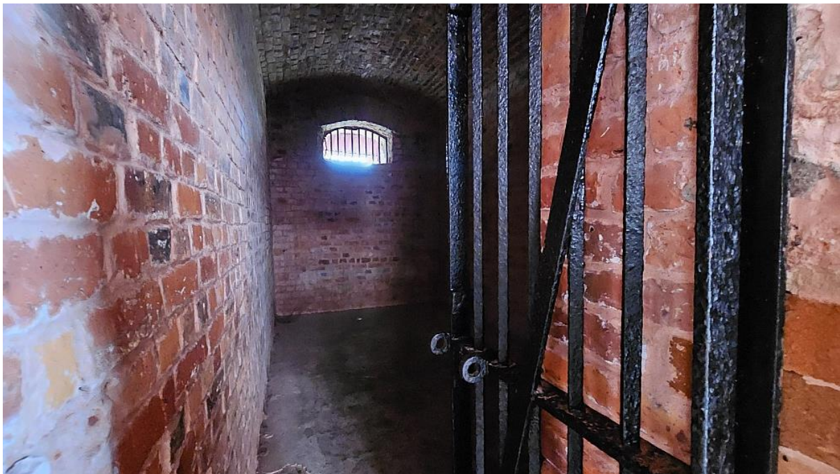
The jail was engineered to provide a more severe and controlled environment than others
