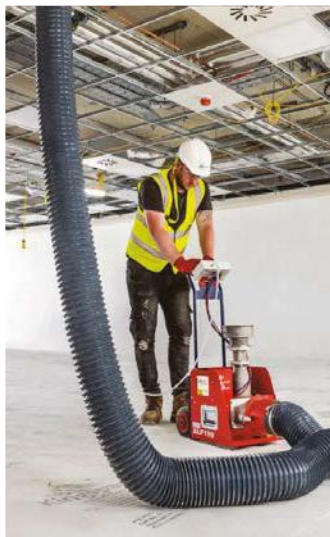
▼ It is therefore of utmost importance that new ductwork is tested soon after being installed.
